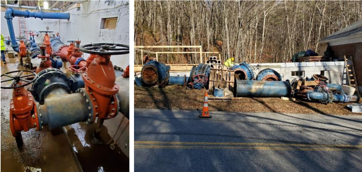
Figure 3 - Narrows Road PRV replacement
