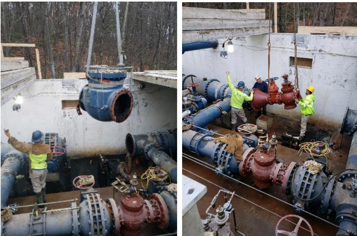
Figure 2 - Installation of PRV
