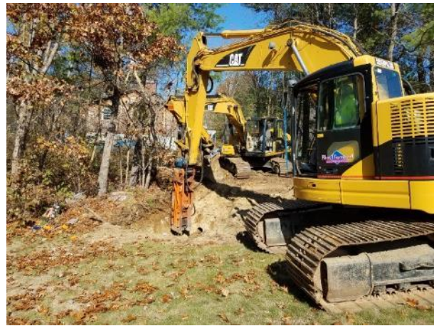
Figure 5 - Contractor hammering ledge, at #110 Highview St
