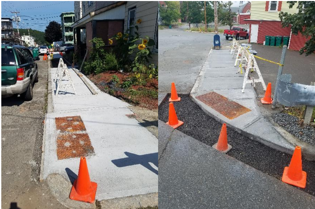
Figure 2 – Clarendon Street and Daniels Street Sidewalk Repair
