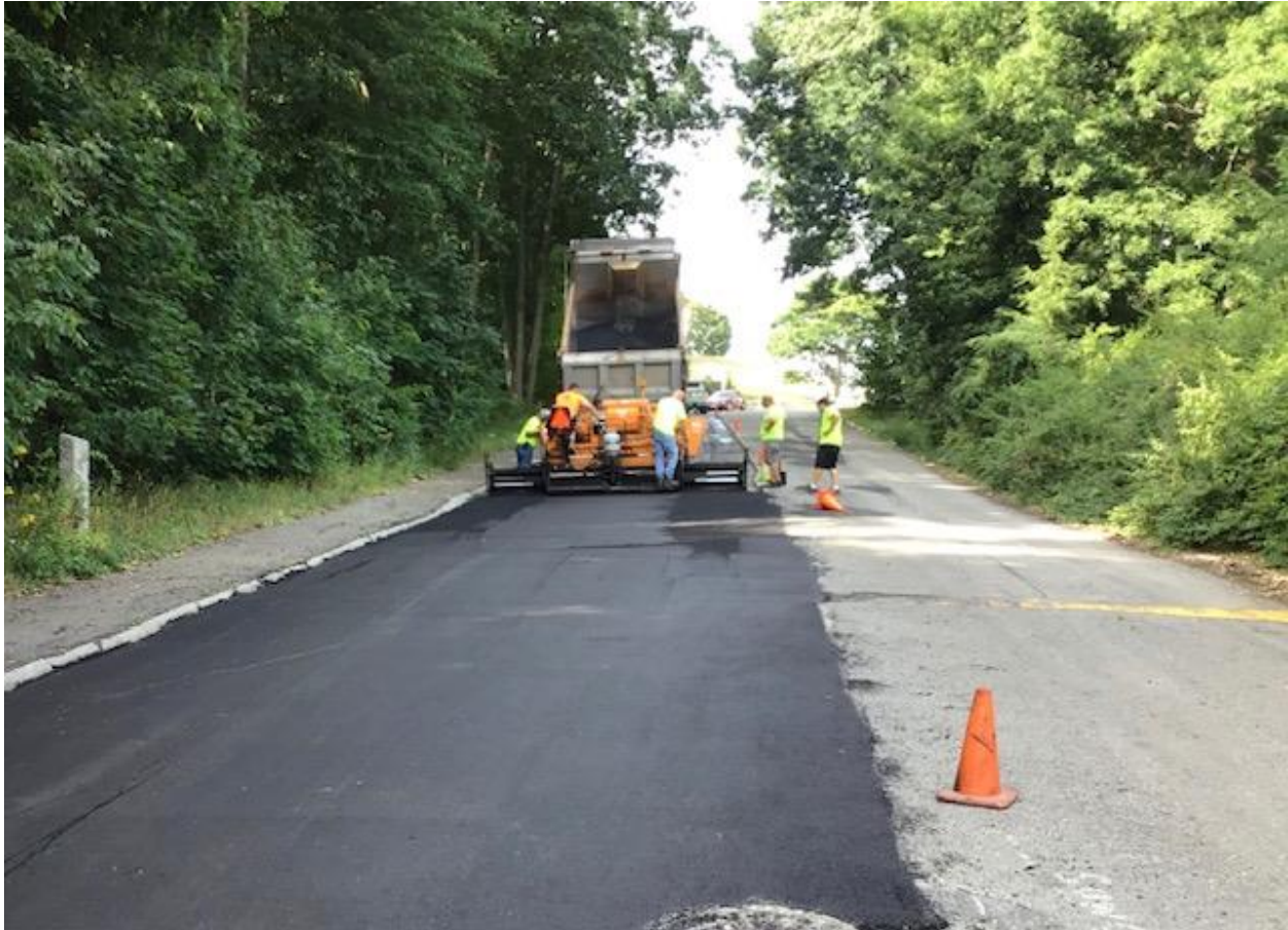
Figure 1 – DPW Paving Meadowbrook Lane
