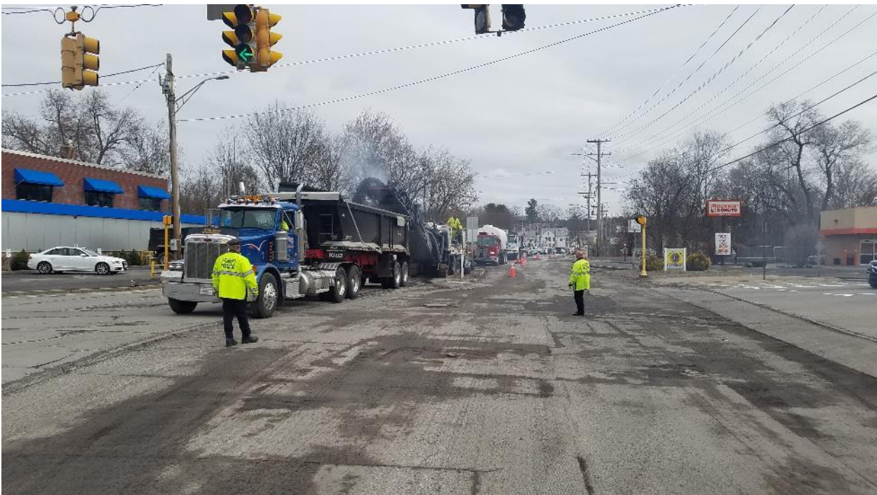
Figure 2 – Lunenburg Street milling in preparation for paving
