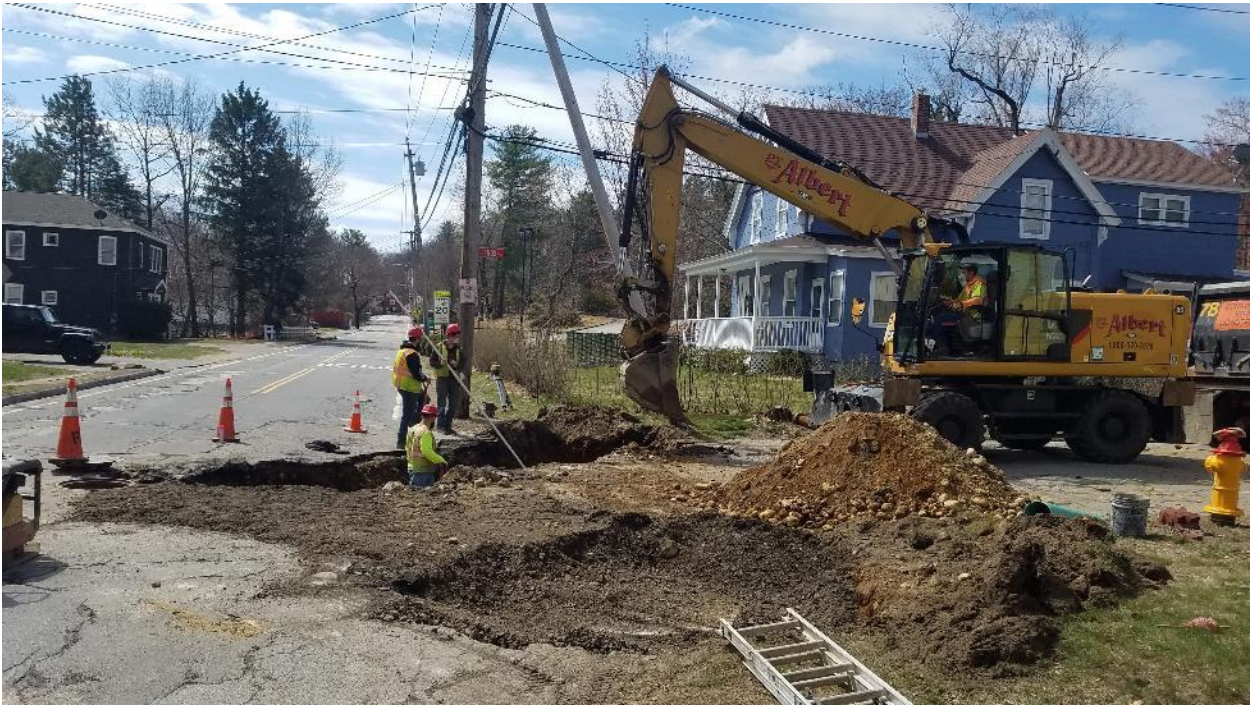
Figure 1 - Installation of CBs at Lenox St
